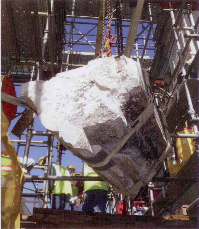
The original granite that was removed to make way for the installation of GFRP panels on the project (shown here) will be recycled.
